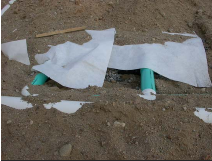
Figure 4: Perforated Pipes (covered by a geotextile fabric) in a Traditional Soil Absorption Bed (Note the gravel seen between the pipes.)
