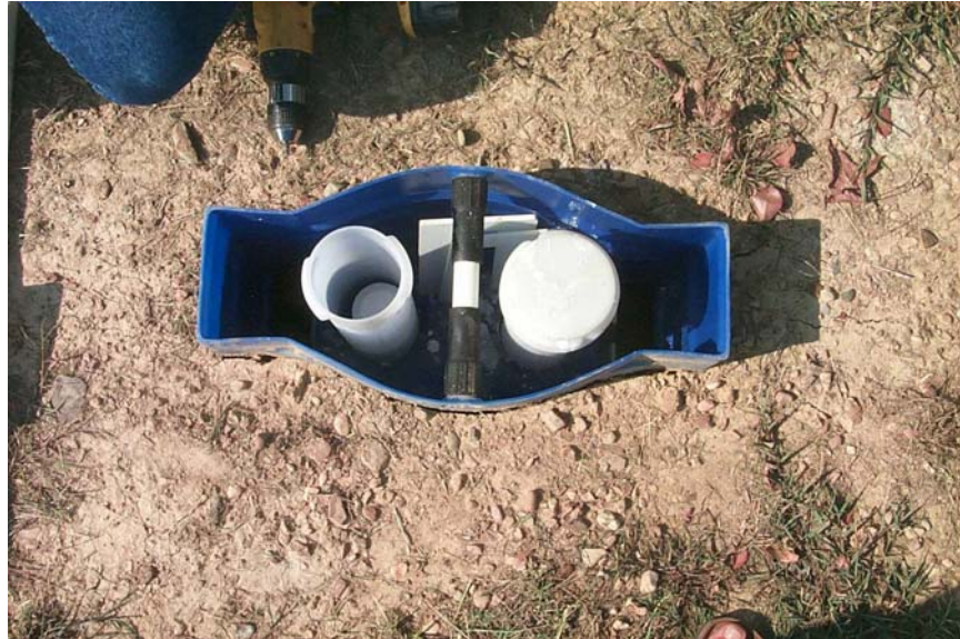
Figure 5 Tablet Chlorinator with lid removed
