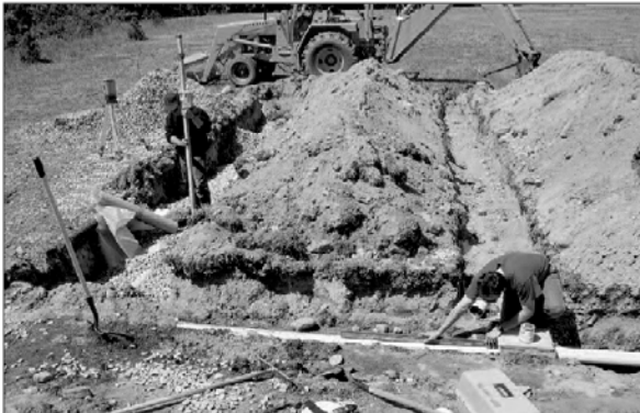
Typical Septic System Replacement Installation
